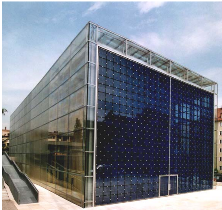
Figure 1 – Glass Façade of Herz Jesu Church, Munich
